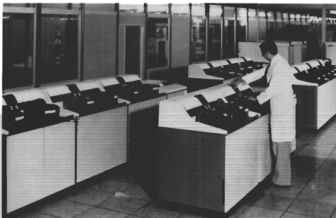
The Olivetti data center in Ivrea, near Turin, Italy, utilizes extensive Memorex equipment including 3675 disc drives and controllers, three 1270 Terminal Control Units, and a Computer-Output-Microfilm System 1600.
